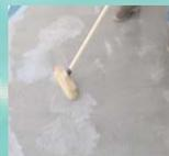
If the slab is too porous (time <60 s): apply a first highly diluted paint coat in order to saturate the concrete slab or apply the appropriate primer.
